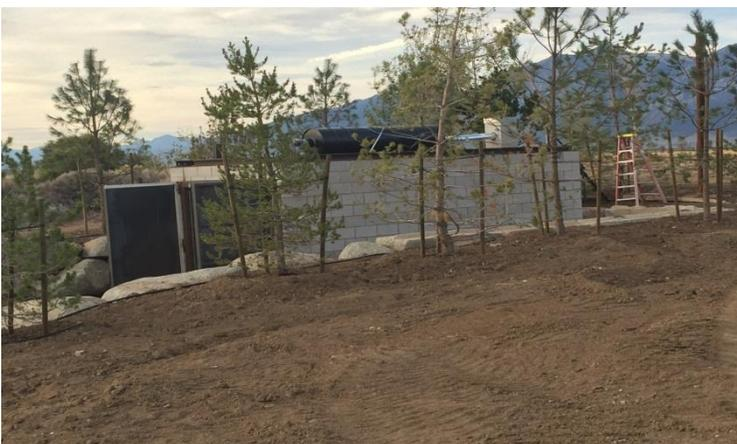
**Photo 3:** Shows Genoa Tree's stationary block kiln in Minden. The kiln is near completion and can process up to 9 cords of chips or whole wood per burn once complete.
